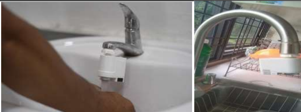
Use of water-saving faucets at the USU Integrated Research Laboratory and the USU Information Study Center
