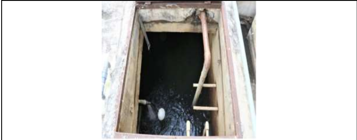
Use of Water Tanks Equipped with Balls (Automatic Buoys) at the USU School of Public Health
